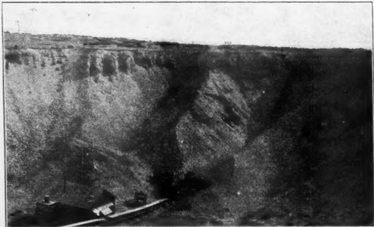
Another View of Pit, Bunker Trap and Conveyor
